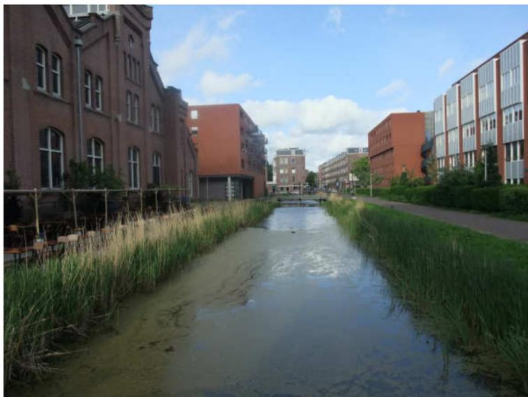
Rainwater capture on the site. About two thirds of the inner area is unpaved; rainwater is directly absorbed here into the ground and does not need to be removed. On the paved parts of the site, the rainwater is not lead to the sewer, but is stored in Waterleliegracht. The canal has an overspill to the Haarlemmer trekvaart (canal) on the other side of Haarlemmerweg. This limits the load on the sewer and surface water.
